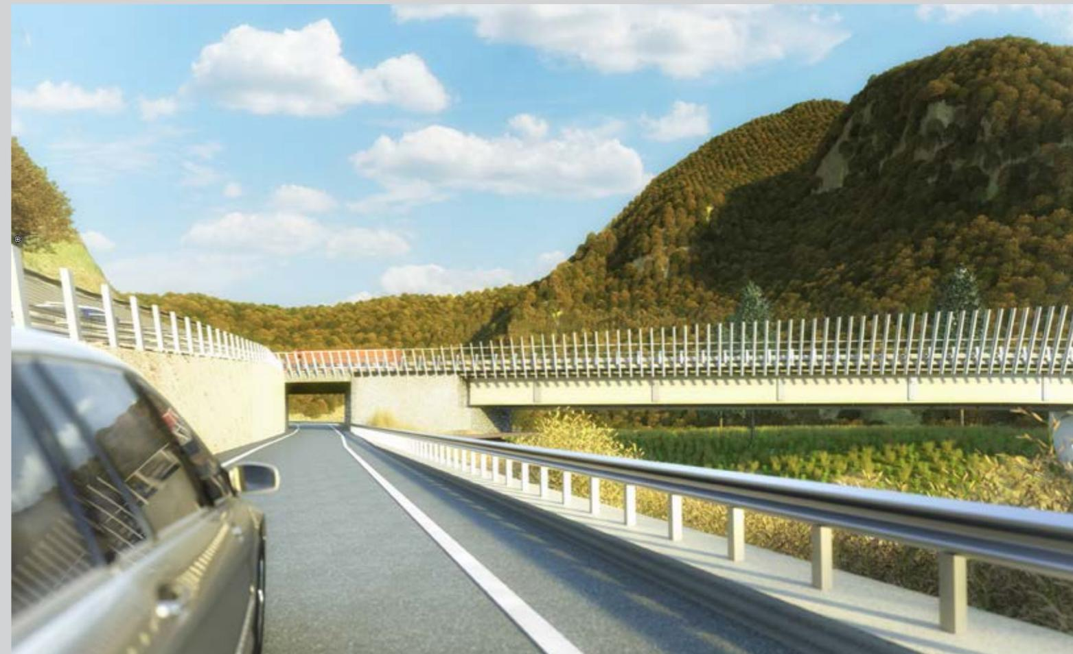
Project for the new motorway on the outskirts of a lake in Northern Italy. One 2 km long tunnel, one 260m bridge, 4km of re-designed surface roads and related works (trenches, embankments, cut&cover).
